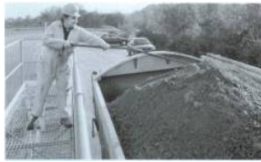
Most sheeting platforms are simple drive-through systems providing a guardrailed platform on each side of the vehicle(Fig. 9)
