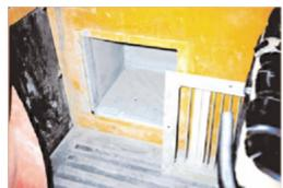
Seating should be capable of being cleaned to prevent build up of dust from overalls.
