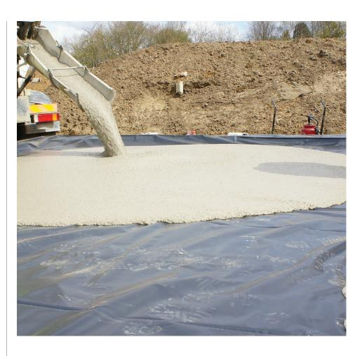
This installation method both reduces the possibility of entrapping additional air within BREEDONFlow Form and eliminates the potential for material segregation due to free-fall around the reinforcing steel and form hardware. Pumping should provide a continuous even concrete rise rate within the formwork with as few breaks in product delivery as possible.
