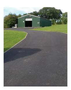
A single layer application also reduces the risk of delamination and potholing by eliminating the possibility of trapping moisture and/or detritus which may occur with a two course treatment. For demarcation or aesthetic purposes, BREEDONOnecoat Parking can also be supplied as a coloured product.
